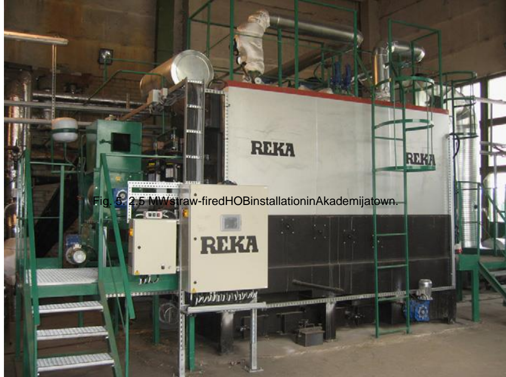
2.5 MW chopped wood fired installation in Akademija town (Kaunas reg.).
