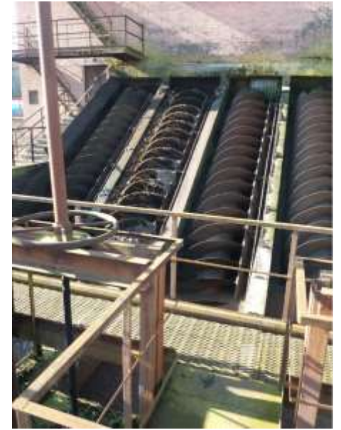
Vilnius WWTP: Archimedes screw pump
