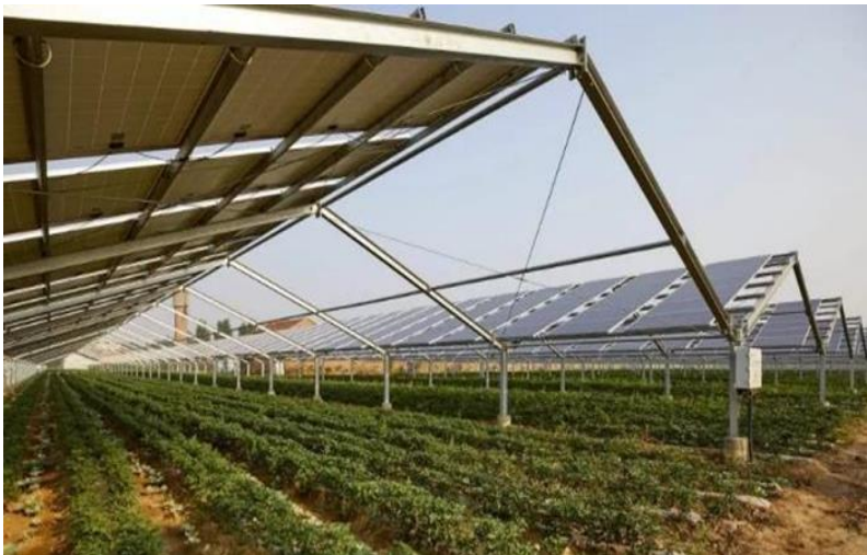
Solar power plant located on agricultural crops
