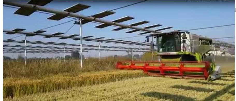
Double-sided photomodules with east-west orientation
