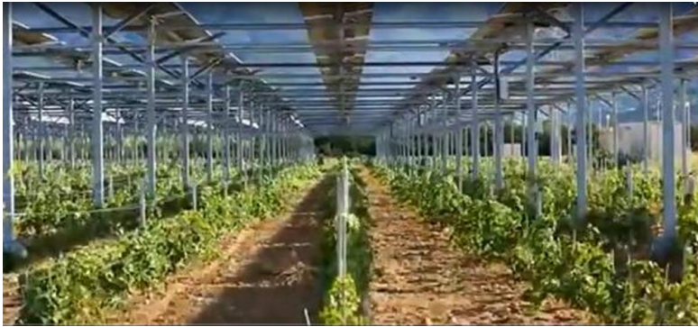
Solar power plant located on agricultural crops
