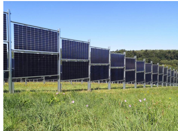
Double-sided photomodules with east-west orientation
